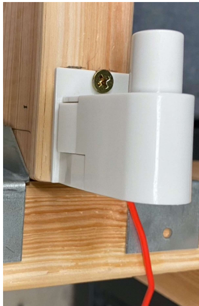
Figure 2.3 Attaching the electrical light socket.
